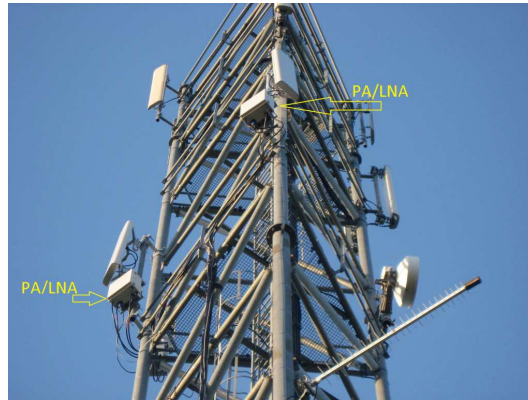
Figure 7.2: Antennas with PAs on mast
