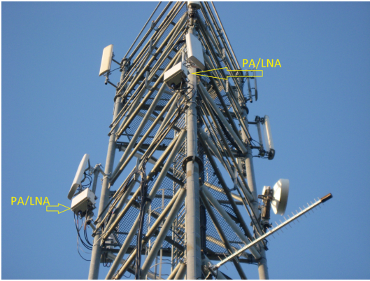
Fig. 2. Antennas with PAs on mast
