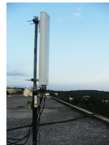
(b) Powerwave Antenna
