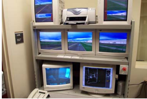
Figure 5 Control Room of the Driving Simulator
