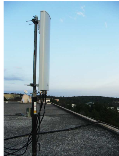
(b) Powerwave Antenna.
